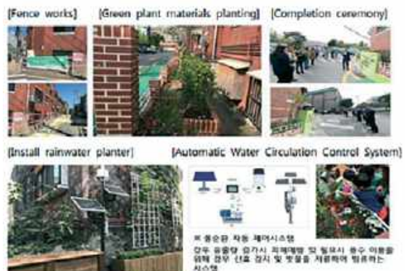
※ Automatic Water Circulation Control System A system for detecting rain signals and detaining rainwater in order to prevent damage and utilize water if necessary when the outflow amount of rainfall is increased
