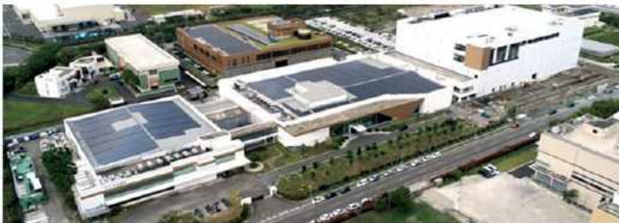
TCI installed solar panels on the rooftops of all factories to self-supply renewable energy.
