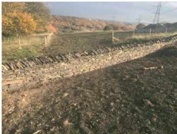
YW641 and 042 Access, 25m of wall removed and reinstated
