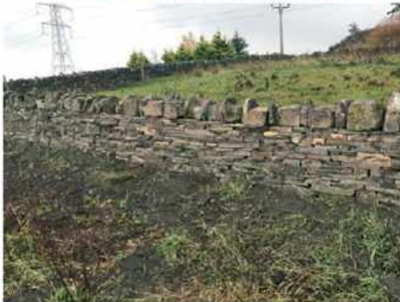
YW047 access, 16m of wall removed and reinstated
