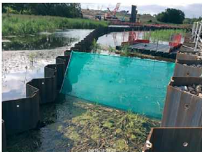
Fish Trap installed at Springhead Bridge
