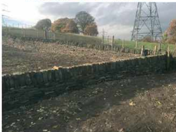
YW641 and 042 Access, 25m of wall removed and reinstated
