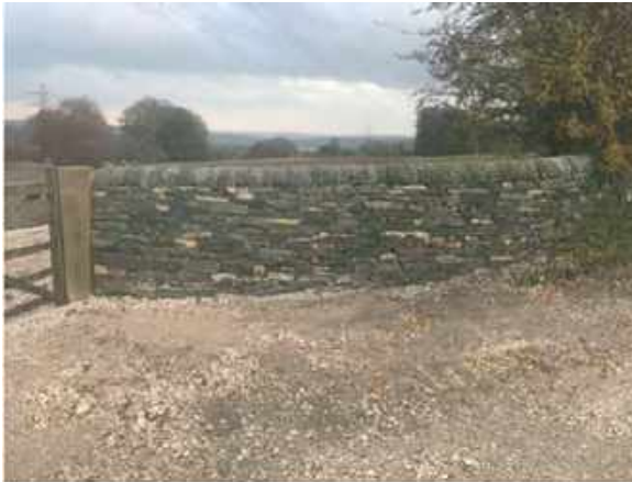
YW047 access, 16m of wall removed and reinstated
