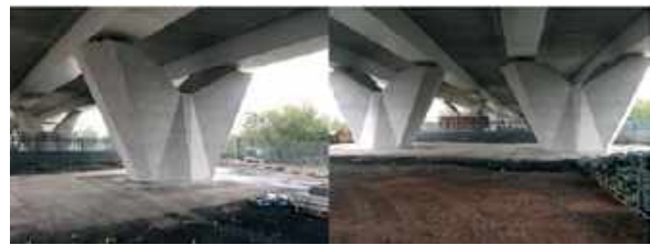
Figure 5 - Photos of completed reinforced concrete jackets
