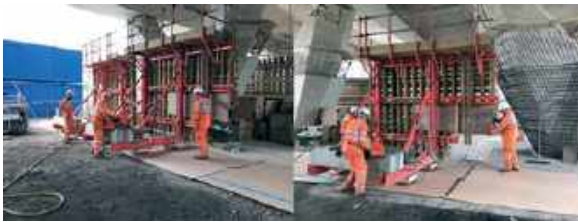
Figure 3 - Use of the air skid to reduce manual handling and plant movements
